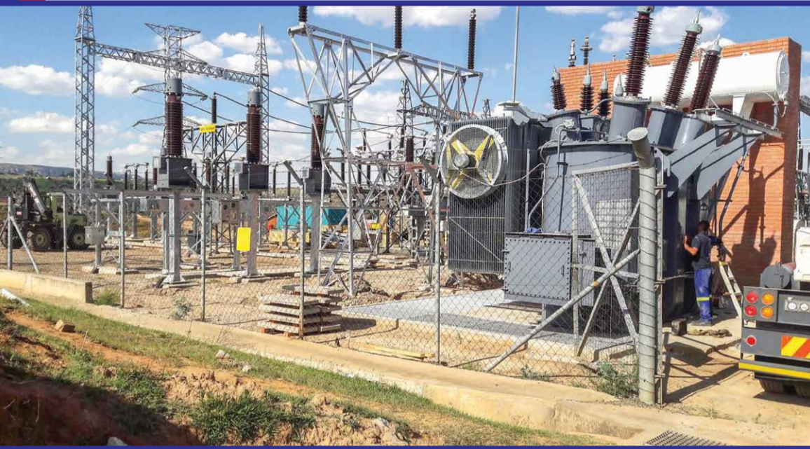
LEC power station
